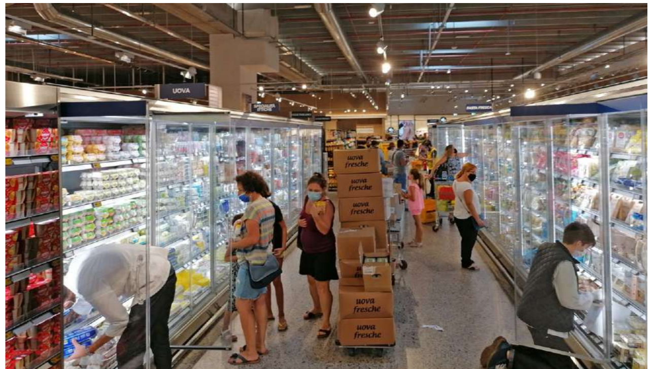
A view of refrigerated space (with energy saving doors)
