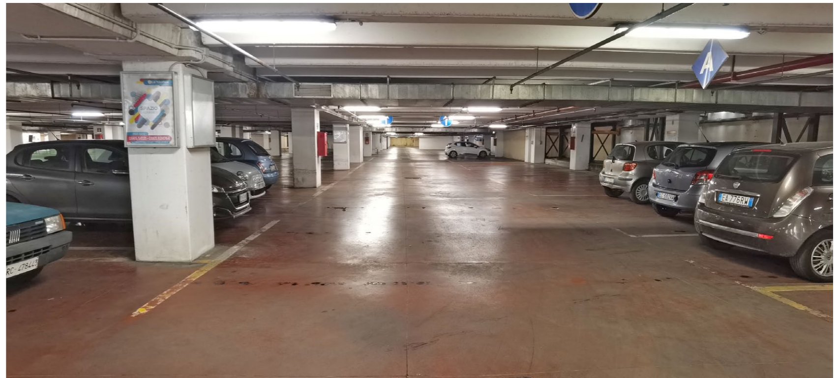
View of the large underground car park
